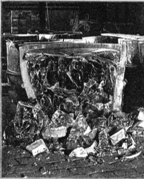
A Cooled Pot with cracked Raw Glass
