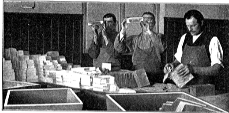
Testing the Glass Slabs
